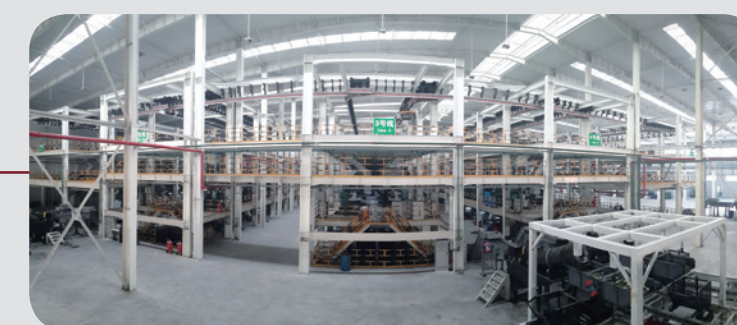
Threading, Air Pressure Test, and Anti-rust Treatment
